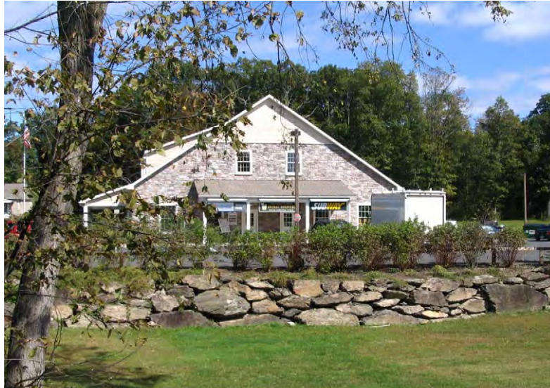
Along Route 209 in Marletown, a commercial building that houses several businesses uses traditional architecture and building materials.
