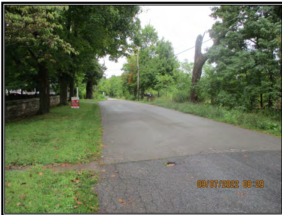
Photo No. 6 – View looking north along Huguenot Street at connection valve location for new watermain
