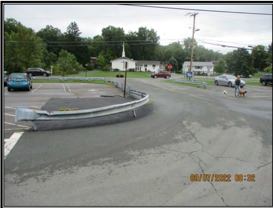
Photo No. 10 – View of connection location on Old Kingston Road toward Route 32
