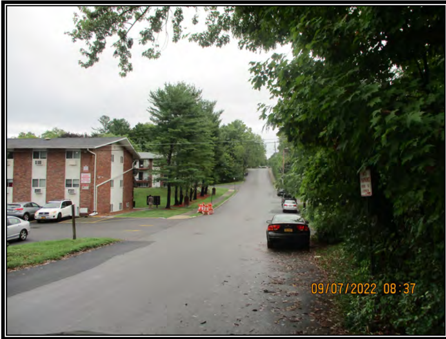
Photo No. 11 – View looking easterly up Southside Terrace toward Route 208 connection location
