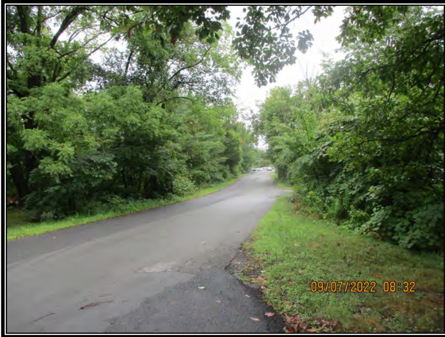
Photo No. 9 – View northerly along route for Huguenot Street Old Kingston Road connection
