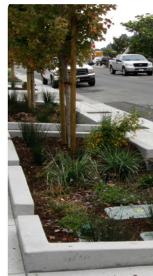
Aesthetically Pleasing Green Practices that Promote Infiltration, Detention and Uptake of Stormwater
