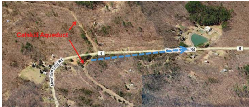
Figure 1: Catskill Aqueduct and New Paltz connection at Mt. Rest Rd.
